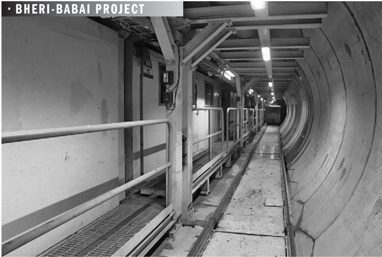
An under-construction tunnel of Bheri-Babai Diversion Multipurpose Project, in Surkhet, on Wednesday.
